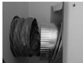
(a few Small 9/16” Screw can be used to affix the flex to the mount)
