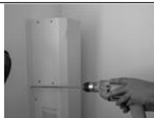
Apply the four plastics anchors on the wall with the help of a hammer.
